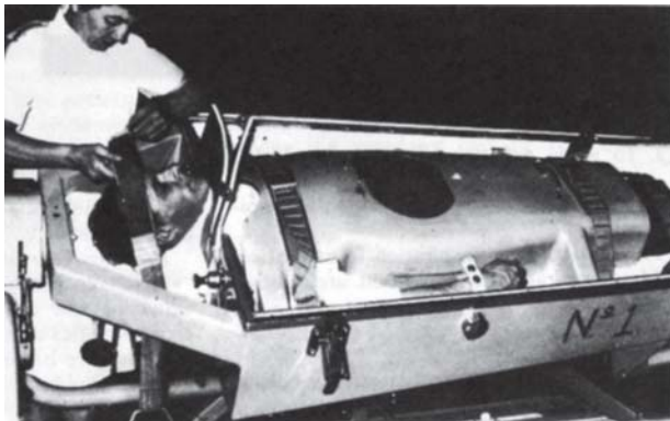
Fig. 2.7: A patient in a rotating iron lung
